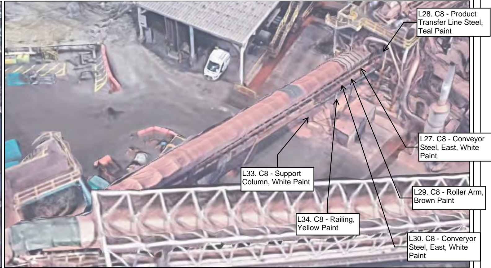
CONVEYOR 8 FACING NORTHWEST
