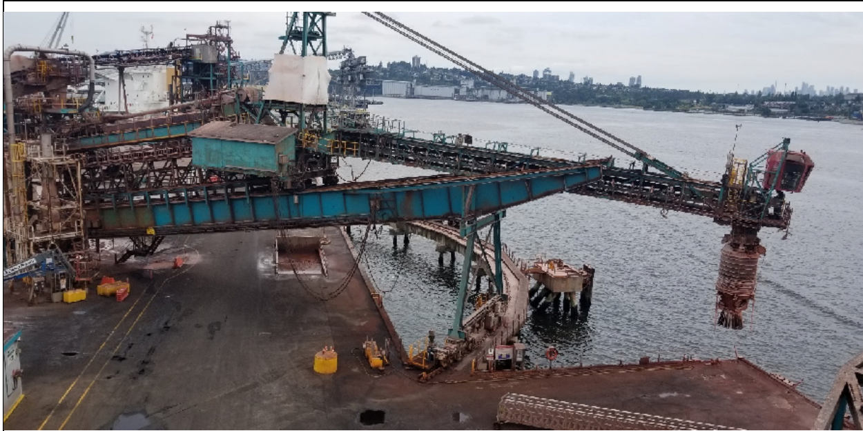
Photo No. 1. Date: 2021-JUL-7 Direction Facing: East Description: View of EPSL and the east quadrant beam from the west.
