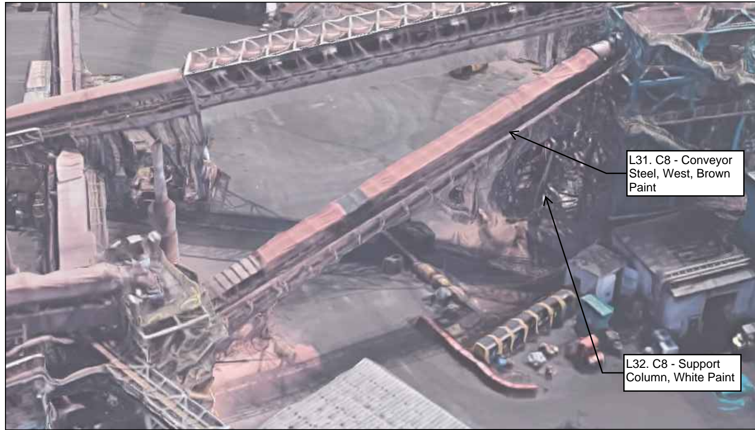
CONVEYOR 8 FACING SOUTHWEST
