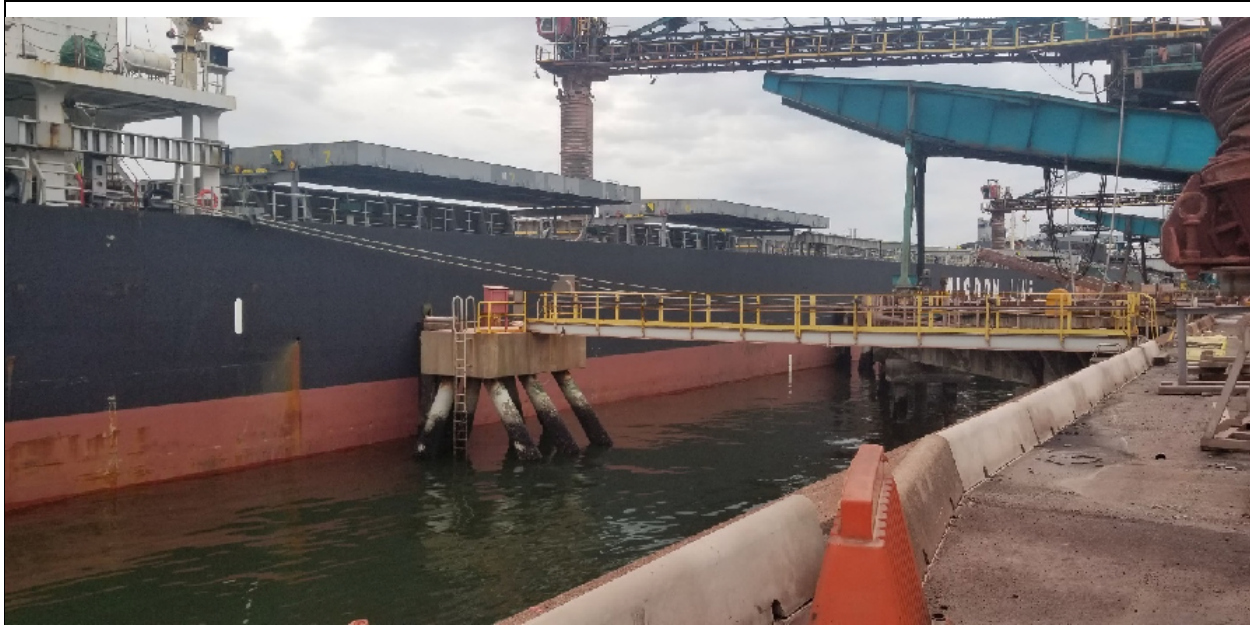
Photo No. 29. Date: 2022-JUN-1 Direction Facing: N/A Description: View of Dolphin 1, with suspected creosote treated lumber support piles.
