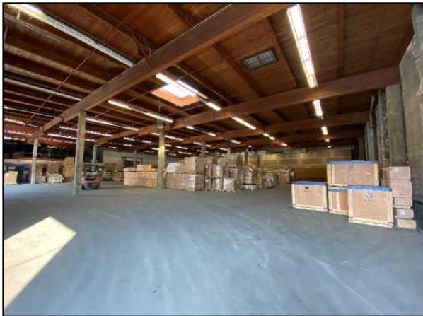
Photo 7 Interior of main warehouse on the property. (2022-10-18)
