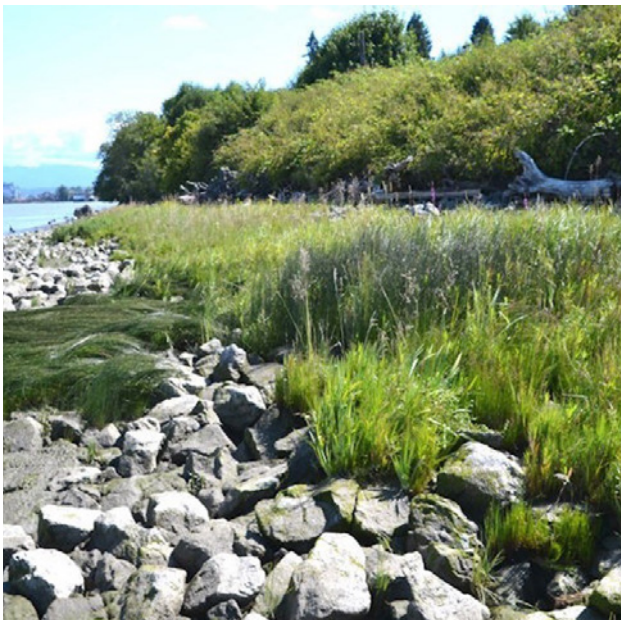
Site conditions at Gunderson Cannery (2021)
