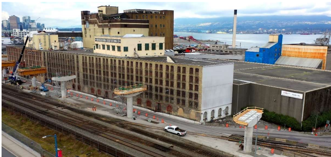
New land on the western expansion is now visible. pre-load material (sand) is being pushed around to the north to infill this area which will become part of the terminal footprint. Phase two pre-load is ongoing.
