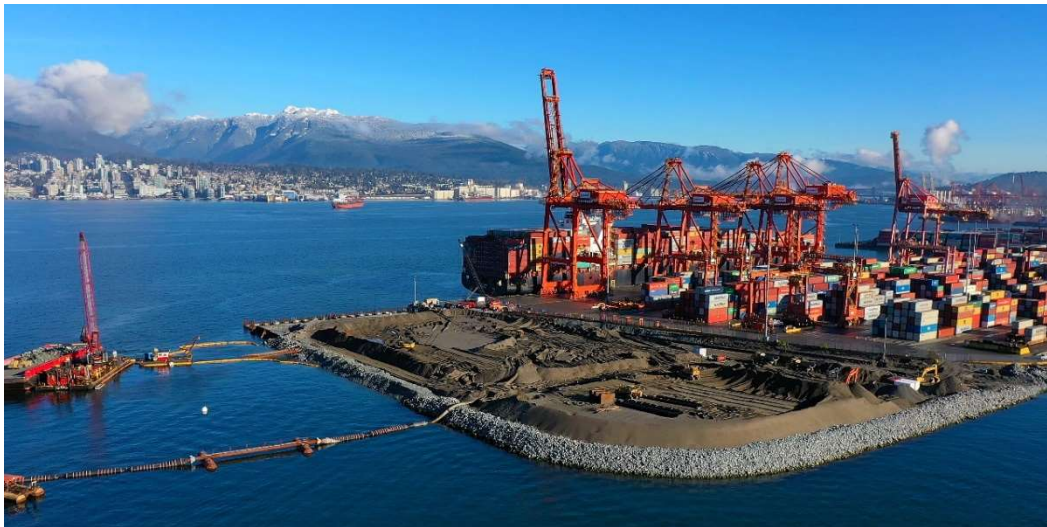
New land on the western expansion is now visible. pre-load material (sand) is being pushed around to the north to infill this area which will become part of the terminal footprint. Phase two pre-load is ongoing.
