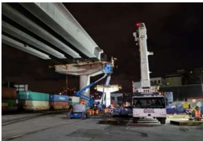
Mobile cranes lift girders into place for the Centennial Road overpass, part of the port authority's Centerm Expansion Project and South Shore Access Project, in February 2021.
