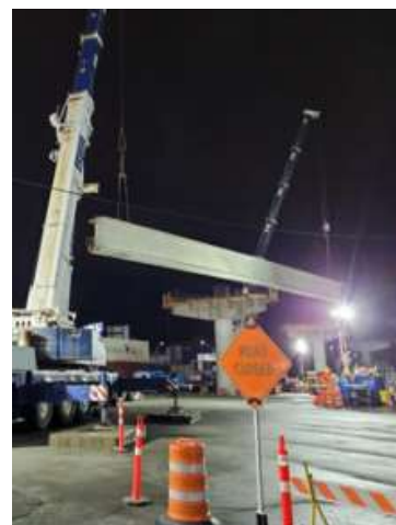
Mobile cranes lift girders into place for the Centennial Road overpass, part of the port authority's Centerm Expansion Project and South Shore Access Project, in February 2021.
