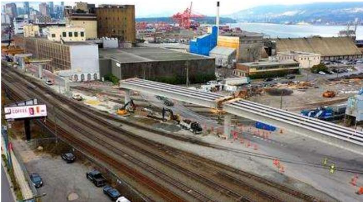
*Pictured: First span of girders installed in early February.*
