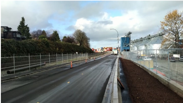
Pictured: Paving completed in front of Columbia Containers
