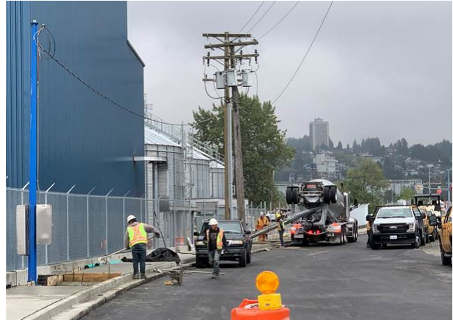
Pictured: Paving the sidewalk near Columbia Containers
