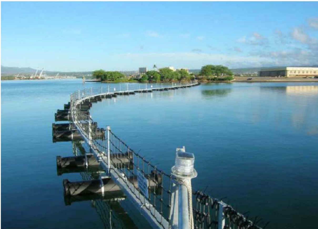
Figure 3: Example of a Similar Boom from an Alternate Installation
