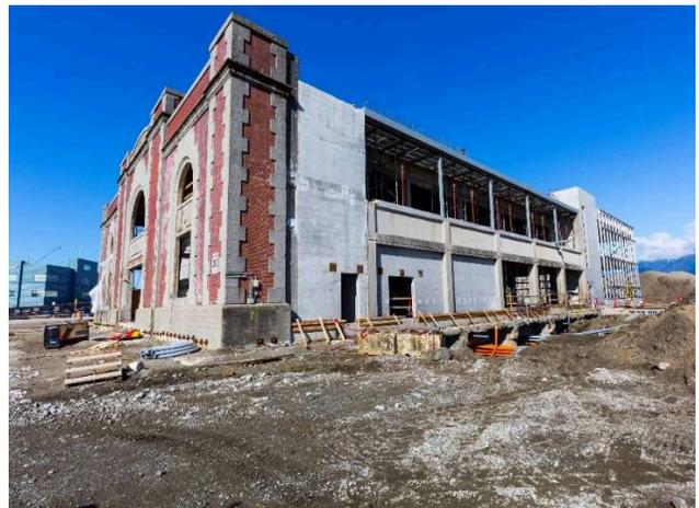
*Pictured: The concrete for the roof of the container operations facility has been poured and the walls of the building are going up*
