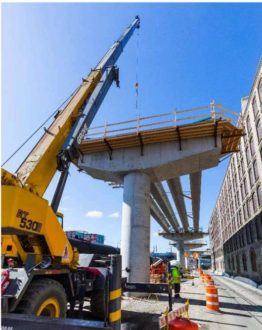
*Pictured: Looking up at the recently installed girders for the Centennial Road overpass*
