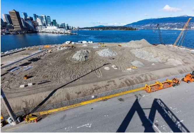
*Pictured: The new rail beams for the rail mounted gantry cranes are visible on the left side of the photo*
