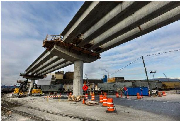
*Pictured: Looking up at the first span of girders for the new overpass that were installed last month.*
