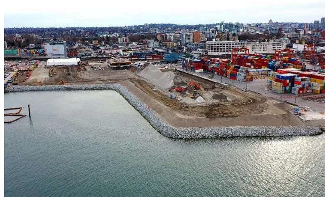
*Pictured: Aerial view of the eastern expansion area. Ballantyne Pier has been entirely demolished and filled.*
