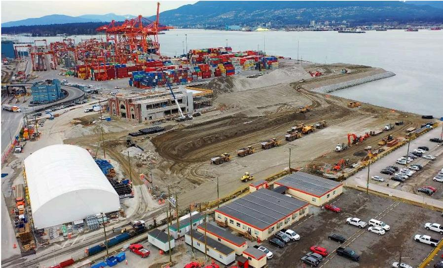
*Pictured: Preload in the eastern expansion area has fully settled and trucks can be seen moving infill to the area around the perimeter of the original Ballantyne Pier.*
