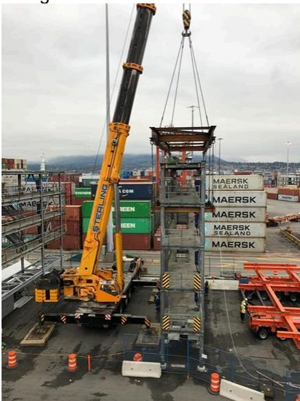
*Pictured: An impressive 500-ton crane lifting one of the refrigerated container towers onto its new foundation.*
