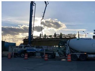
*Pictured: Concrete pour for the beam happening onsite.*
