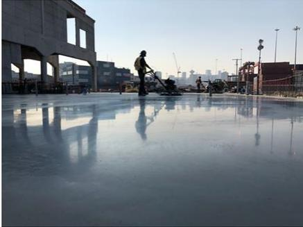
*Pictured: Concrete slab levelling on the bottom floor of the new building.*
