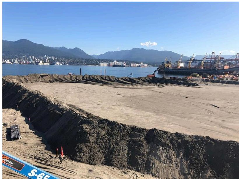
Earlier this month, the Fraser River Pile and Dredge 309 dredging vessel (FRPD 309) returned to the project site to complete infilling in the lagoon in the eastern expansion area. The first phase of the
