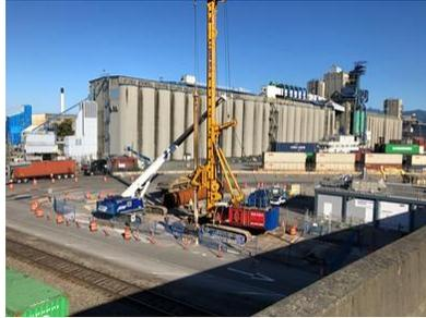
*Pictured: Drill rig for piling work on new overpass.*
