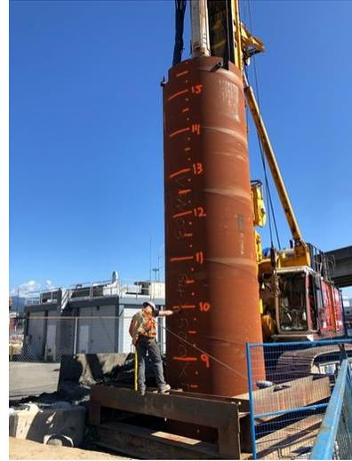
*Pictured: Casing for pier shaft on the new overpass.*
