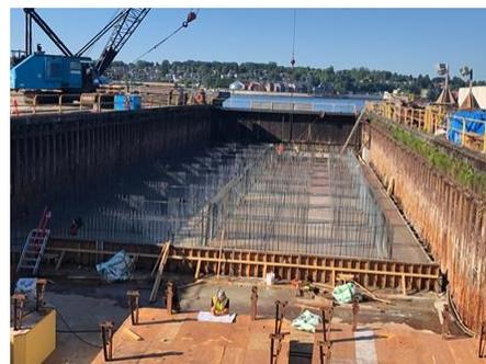
Building a caisson involves pouring concrete into a continuously moving form "slip form". This construction method allows for rapid and economic concrete pouring to build tall or long structures.
