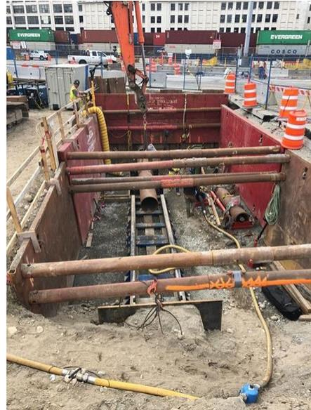
On the project, cables need to be installed across the intermodal yard, which has four rail tracks and two rubber tire gantry crane beams (RTGs). Installing cables is normally done by digging a trench from above, however, when this is not possible an underground tunnel is created to feed the cables through the drilled hole. This is called "trenchless excavation".
