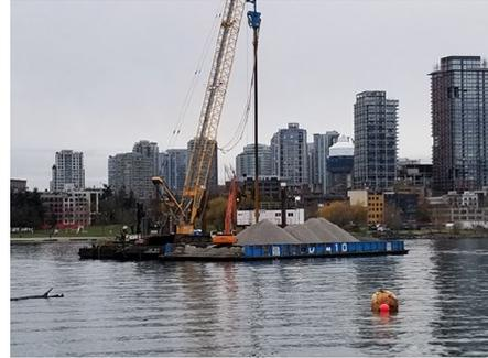
Once the western dykes are built, we will infill behind the west dykes to create new land on the southwest side of the terminal. On the northwest side of the terminal, we will begin densifying the seabed in that area in preparation for the caissons.
