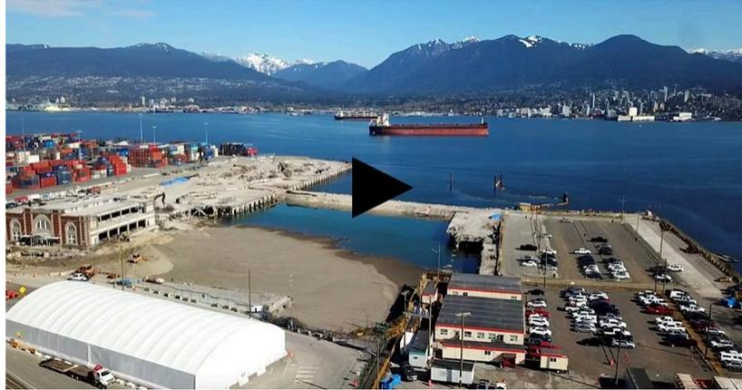
Since January, we've completed dredging and we are currently infilling at the northeast dyke and west end dykes. Here, you can see that the lagoon is now half filled with new land. We have also demolished the old equipment shed and main structure at Ballantyne Pier, and have begun laying the groundwork for the new reefer towers on terminal that will help keep refrigerated containers cool.
