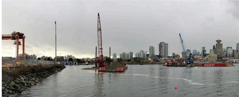
Dredging work on both the eastern and western expansion of the Centerm container terminal was completed last month. Infilling is underway on the northeast corner and west of the terminal. This will allow us to install caissons, which are hollow concrete blocks that are each 20m in height. Caissons are expected to be installed this summer. Infilling in the lagoon on the eastern expansion area is on hold until work can be safely carried out with the lowest risk to fish and habitat.
