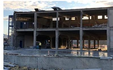
*Pictured: Slab demolition and sorting work at Ballantyne Pier.*
