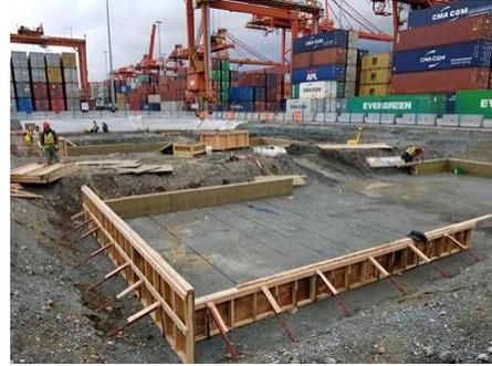
These four structures will accommodate up to 120 containers (standard 40ft equivalent container size), stacked up 5 high. We anticipate that the reefer towers will be up by June.
