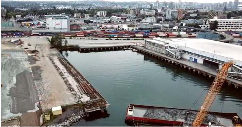
It can be hard to see what's happening on port land from the city. This video gives you a bird's eye view of work happening at Burrard Dock (removal of the rail ties) and a dredging barge with silt curtain in place.
