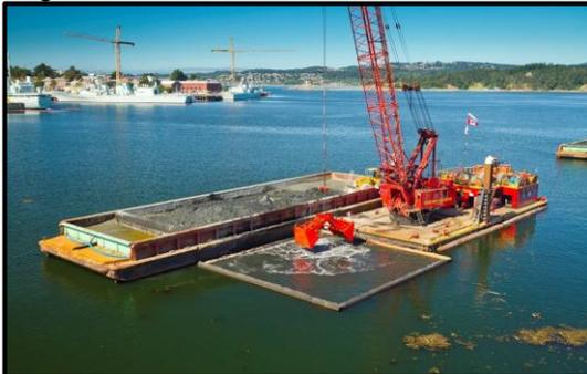
Barge-mounted crane with clamshell dredge, silt curtain frame and dredge barge
