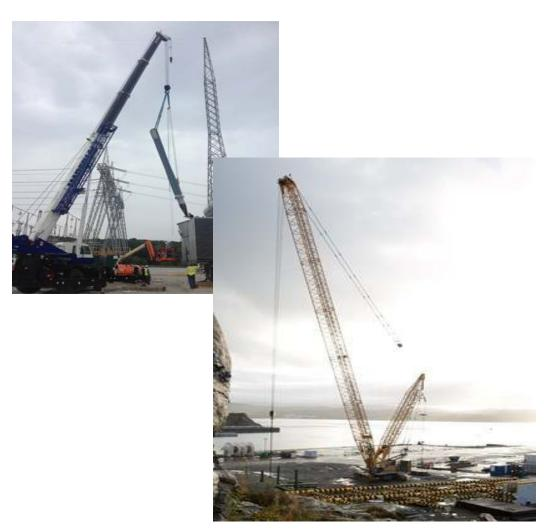
Two cranes will be stationed on-site to load/offload material from barges and trucks in the laydown areas
