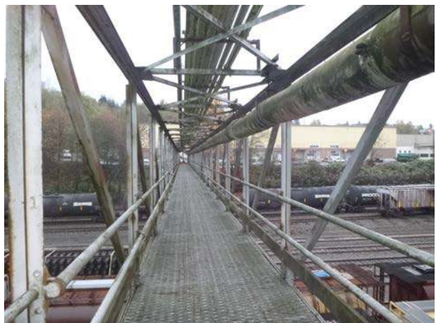
Existing Bridge Showing Utility Transportation
