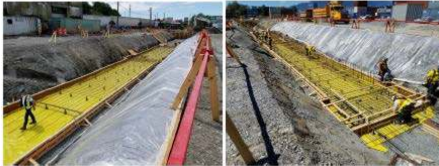
Figure 4 - Installation of rebar for the Reclaim Tunnel Slab Module 04 - June 20 & 21, 2017.
