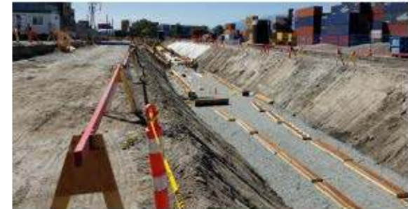
Figure 5 - Installation of Loading Tower Foundation Pedestals - June 20 & 21, 2017
