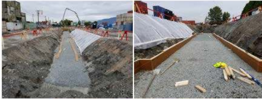
Figure 3 - Installation of Reclaim Tunnel Module 04, 05 formworks - June 17 & 19, 2017.
