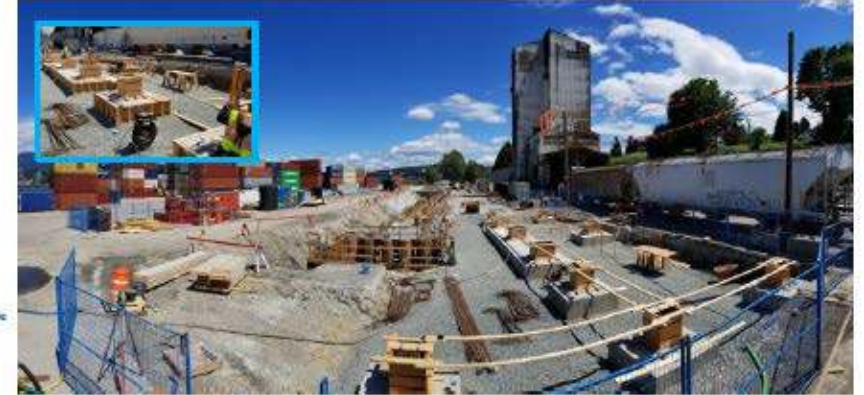
Figure 5 - Installation of Loading Tower Foundation Pedestals - June 20 & 21, 2017
