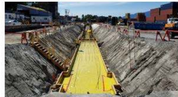
Figure 12 - Formwork Installation for Reclaim Tunnel Module 05 & 06 - June 26 - 30, 2017
