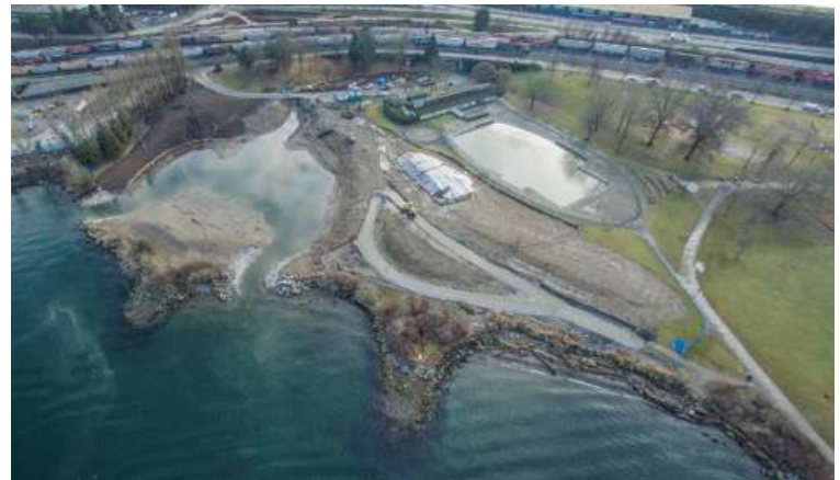
January 2017 (ongoing construction)
