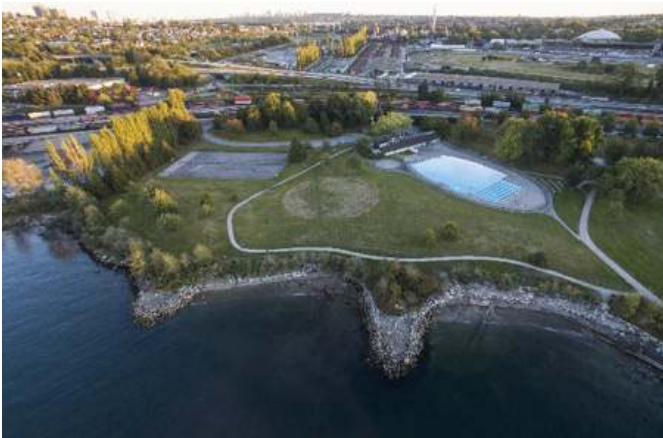
September 2016 (before construction start)
