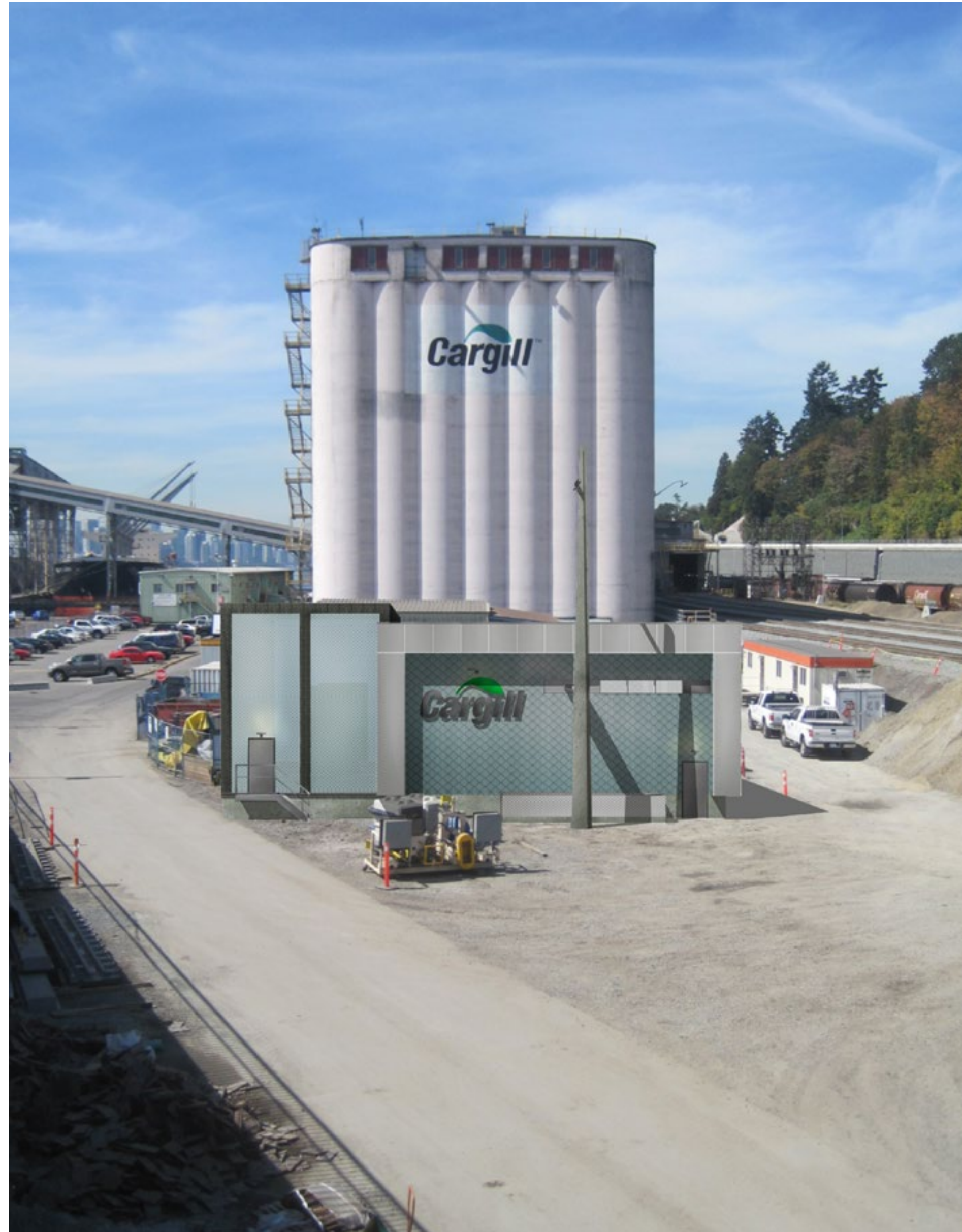
1 A-00 VIEW FROM EAST ABOVE ACCESS OVERPASS
