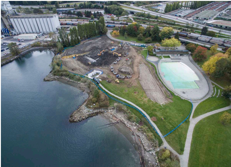
Aerial shot of the construction site at New Brighton Park.
