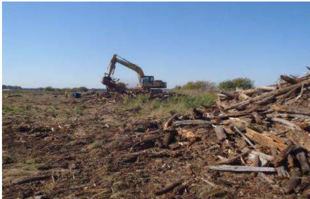
Photo 9. Excavator removing logs from Site 3.3 (September 2013).
