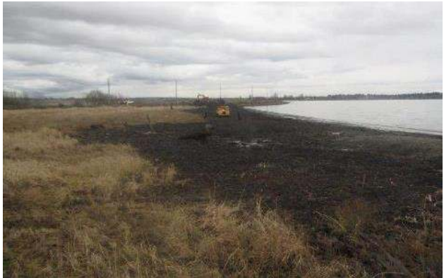
Photo 3. Salt Marsh Restoration Site 3.2 following the woody debris removal works (January, 2014).
