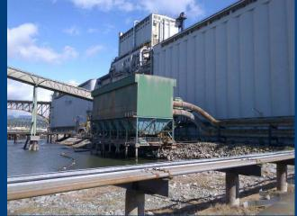
Efficiency of filtration is low by current regulatory standards
