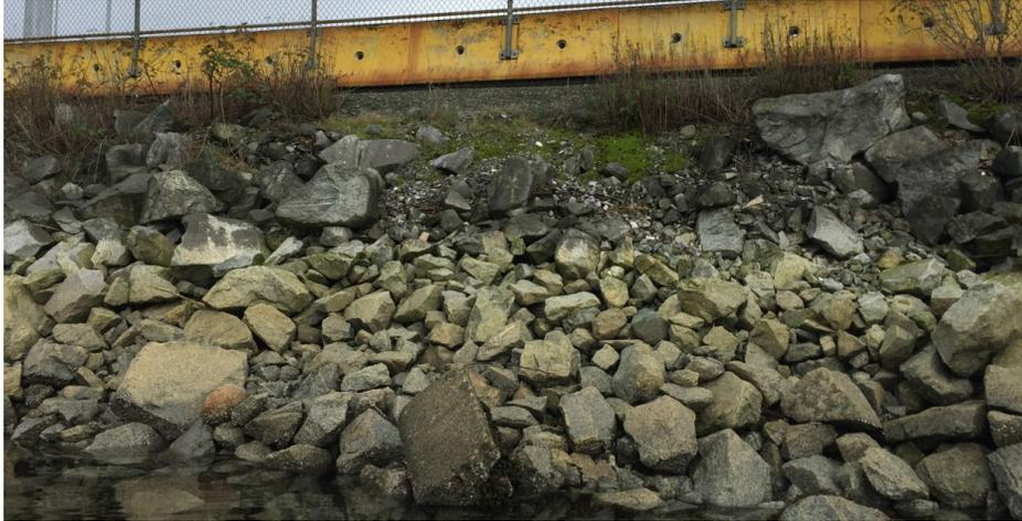
*Figure 3.1: Minor Damage of Upper Crest of a Rock Armour Slope*
