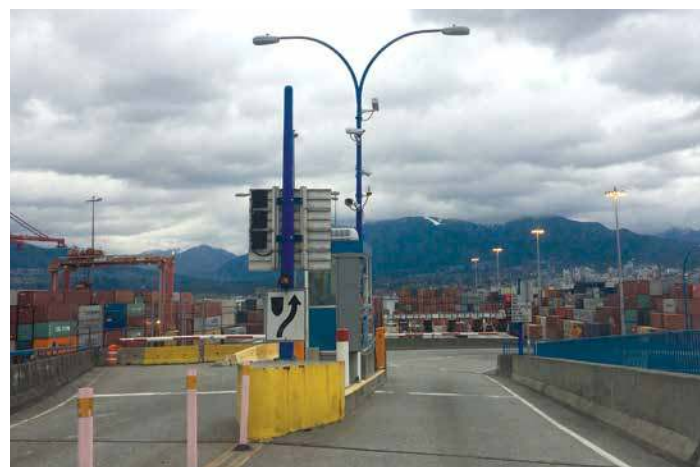
Existing Vehicle Access Control System Gates
