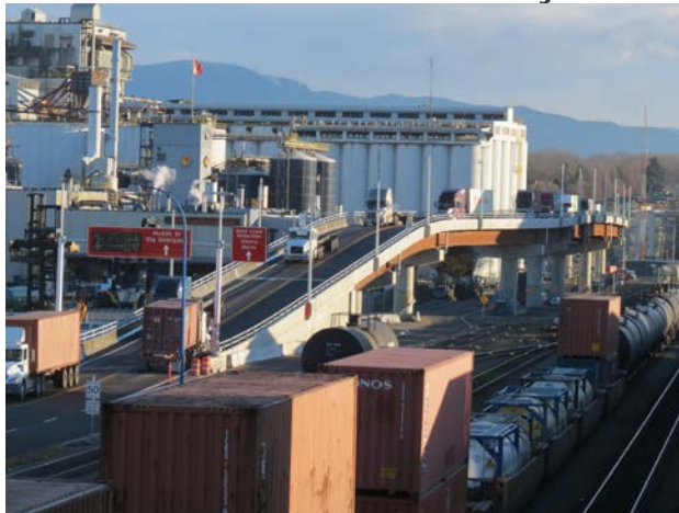
Stewart Street Elevated Roadway
