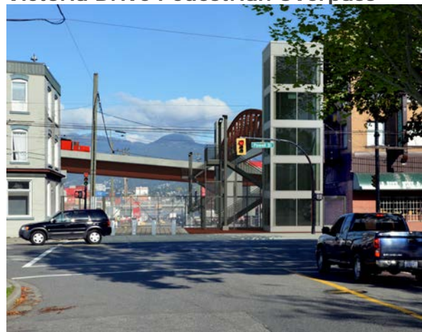
Victoria Drive Pedestrian Overpass
